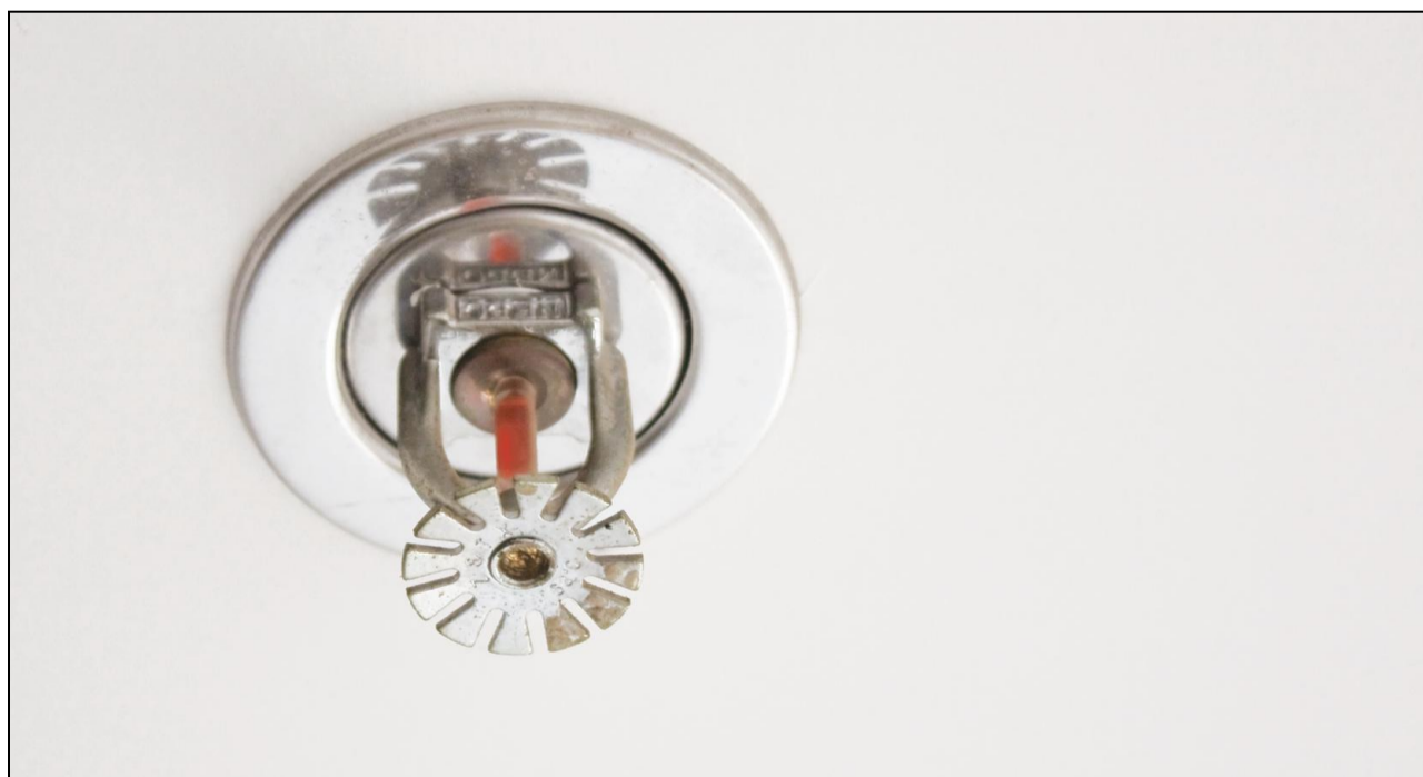
Does it work? If you state that your premises has a sprinkler system installed, it must be in full working order.
